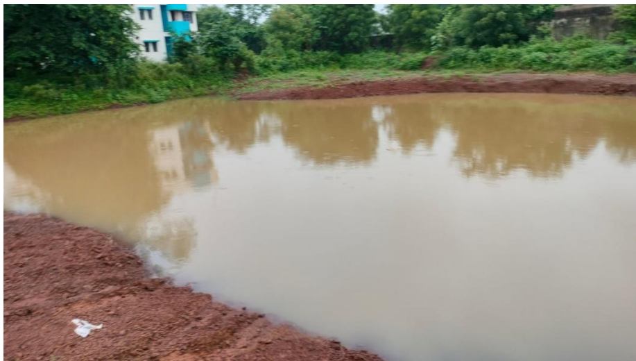
Plate 2: Surface water management
